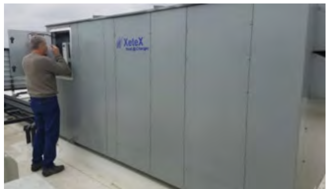
Example DOAS Ventilation Units and Heat Recovery Core
