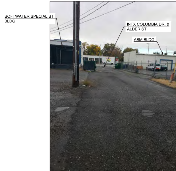
EXTG POWERPOLE AT ALDER ST & ALLEY INTX. (FACING NORTH)
