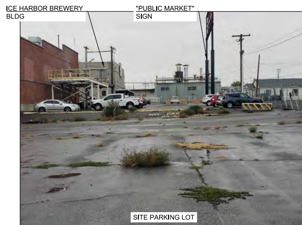
SITE BORDERS ICE HARBOR BREWERY PARKING LOT EXTG ELEVATION CHANGE BETWEEN PARKING LOTS (PROPOSED SITE FACING NORTH TOWARD ICE HARBOR)
