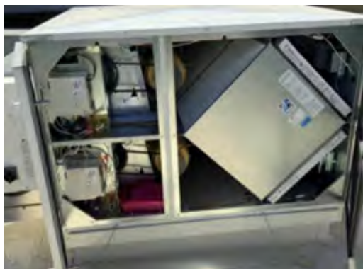
Example DOAS Ventilation Units and Heat Recovery Core
